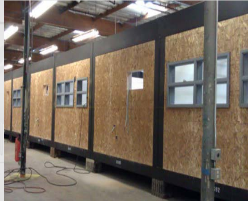
Building shell fabricated off-site
