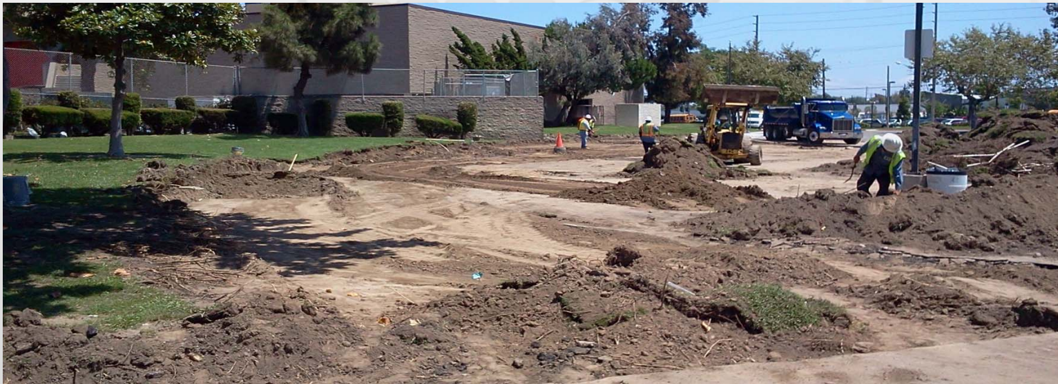
Parking lot improvements
